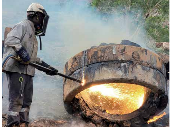
Oxy cutting steel into smaller pieces
