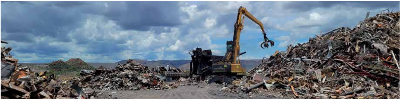
Shears used to cut steel
