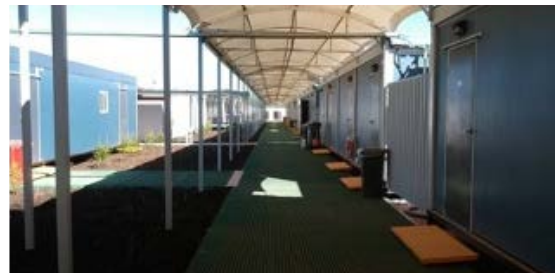
Comparable camp – walkways between rooms
