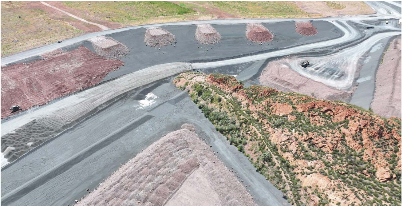
West Dam Embankment rock stockpiles being spread over profiled surface
