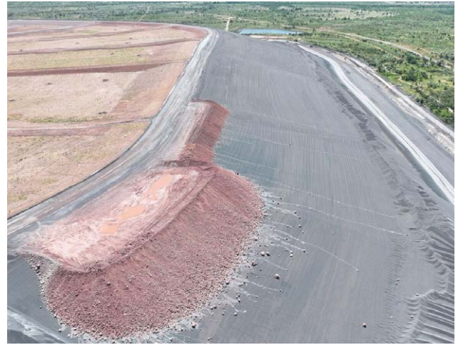
Main Dam Embankment rock armour stockpiling
