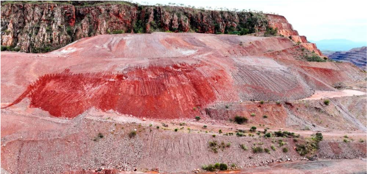
South West Upper (SWU) reprofiling works
