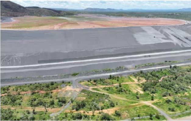
TSF main dam embankment reprofiling works
