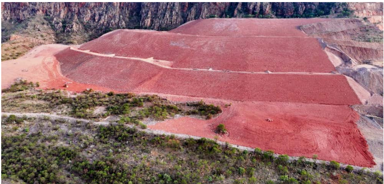
Growth media spreading completed on the SWU
