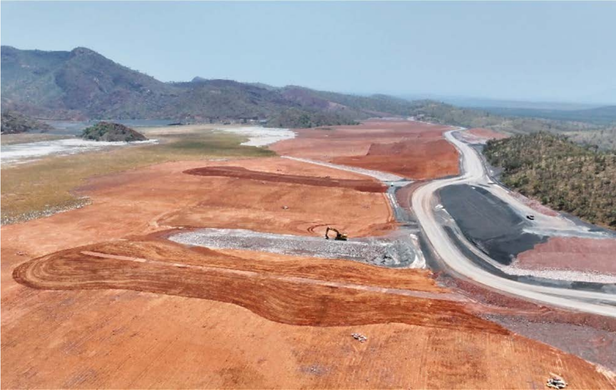
TSF Surface – Growth media ripped and spread
