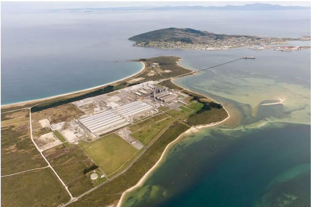
New Zealand Aluminium Smelter, Tiwai Point, New Zealand
