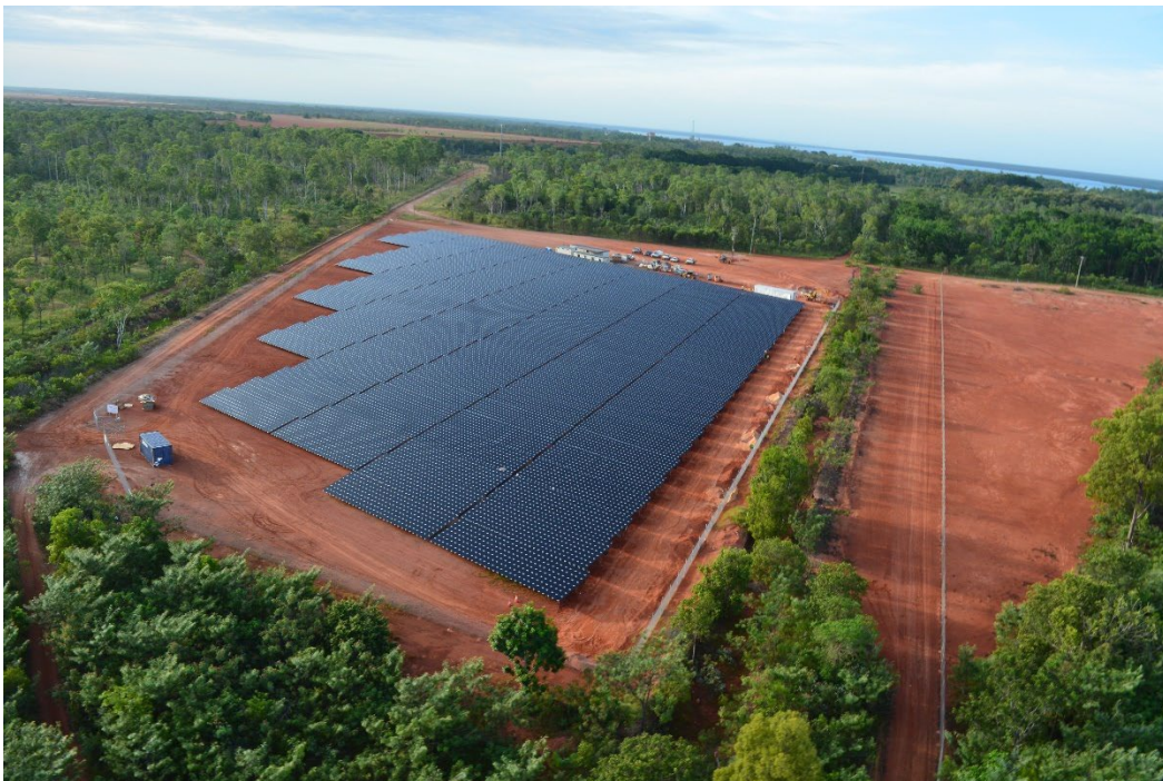
Rio Tinto Weipa, solar panel installation
